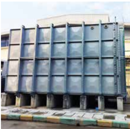
GRP - SMC Panel External Brazing type tank
